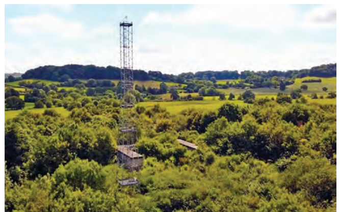
Seen from the air the bunker is not obvious; only the ventilation towers and aerial mast are easily visible
